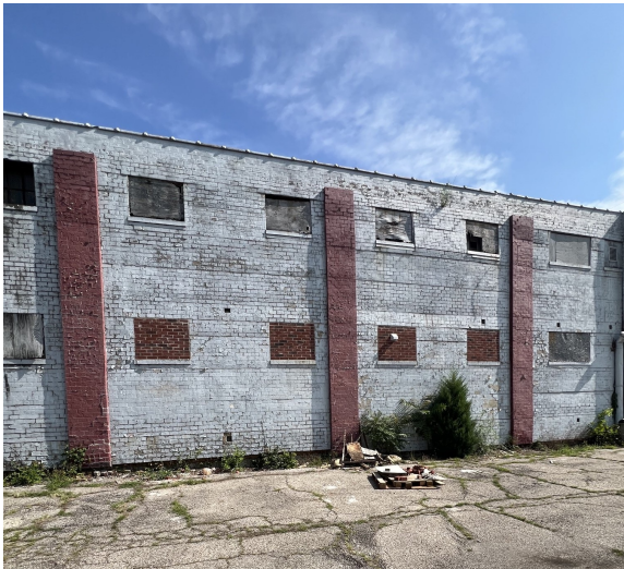
Ground floor windows bricked up
