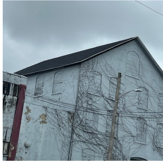
The completed roof repairs
