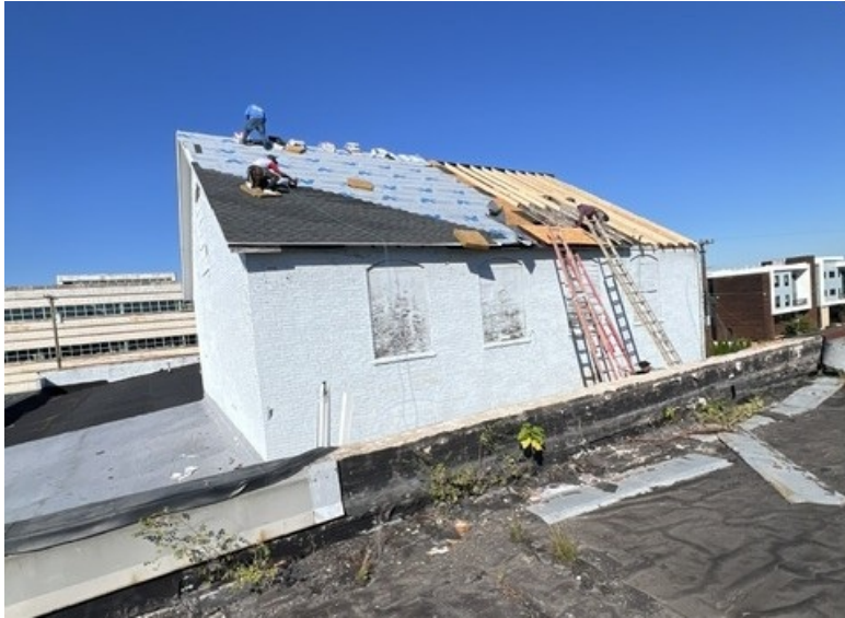
Repairs underway on the roof of BTM
