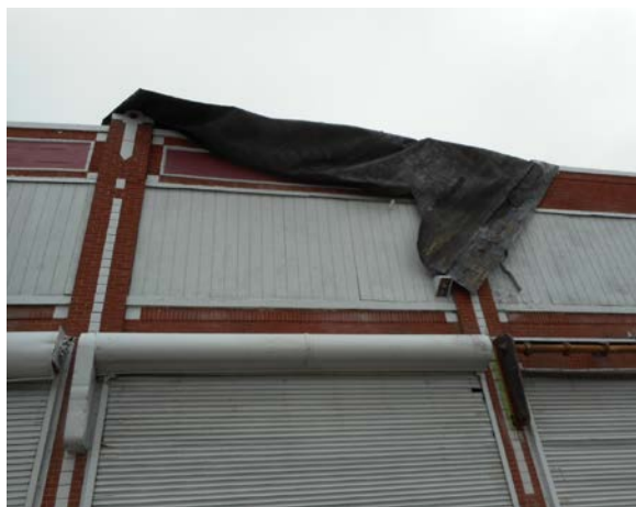
Rubber membrane blown loose on the roof.
