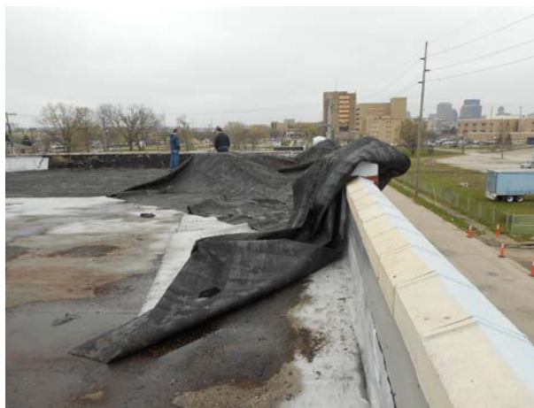
Rubber membrane blown loose on the roof.
